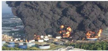
Smoke pours from petroleum storage tanks following a 2009 explosion at the Caribbean Petroleum Corp. refinery in San Juan, Puerto Rico. The blast and fire damaged 17 of the 48 tanks at the site, and flames burned for pearly 60 hours. Photo coursesy of the LIS Chemical Safety and Hazard Investionation Board.
